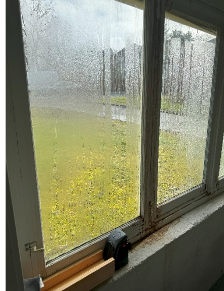
View of the hallway in the dwelling unit. This portion is partially below grade. As seen in the above images, there is lack of insulation, and the windowsill shows signs of water damage.
