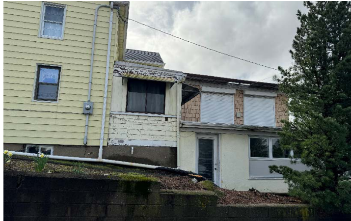
View of the westerly façade of the building from the parking lot to the west. The images show signs of deterioration with visible rust, cracks, and peeling paint.
