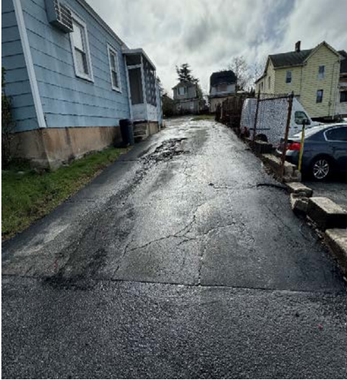
View of the entrance driveway from 11 Church Street. The driveway is narrow and extends up to the property line. Overall, there is a lack of maintenance and signs of disrepair as exhibited by cracks in the driveway and potholes.
