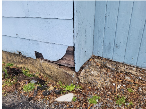
The southerly façade of the residential structure shows signs of wear with deteriorating foundation and cracked siding.
