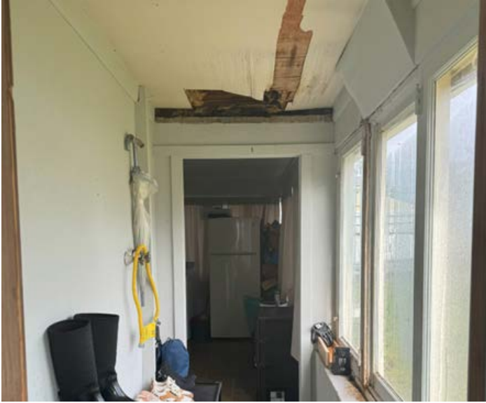
View of the hallway in the dwelling unit. This portion is partially below grade. As seen in the above images, there is lack of insulation, and the windowsill shows signs of water damage.
