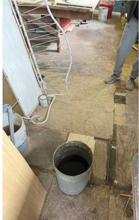
Unfinished flooring with scrap of plywood. Buckets are placed to collect water from the leaking roof.
