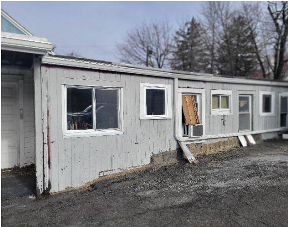
View of the rear façade of the nonresidential use. Exterior siding is worn and peeling. The windows are mismatched with warped frames. Scraps of metal are used to support gutters.
