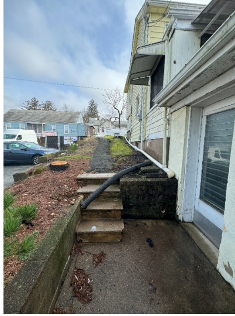
View of the side yard (west) looking towards the rear yard. The walkway shows signs of disrepair. As seen in the above image, the drainage pipes expel rain water on to the side yard that potentially flows on to the street or the neighboring property.
