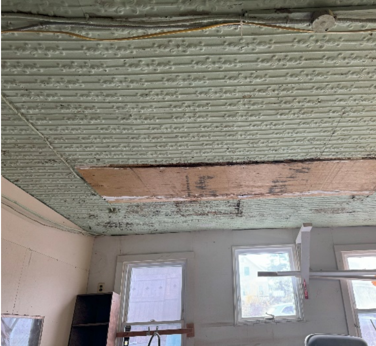
Makeshift repairs to the ceiling panels with plywood. Exposed wiring on ceiling.
